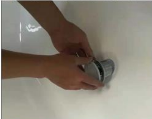
Step 7: Connect the overflow pipe to the waste.
