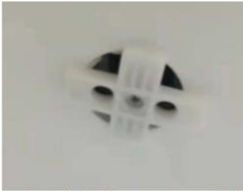
Step 6: Install the replacement waste onto the bath.
