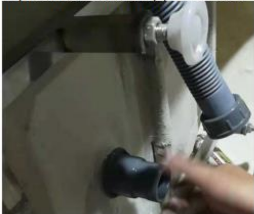
Step 7: Connect the overflow pipe to the waste.
